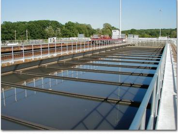
36 ft wide Clarifier - SAV 709 Chain with HMAX Extreme Duty Flights
